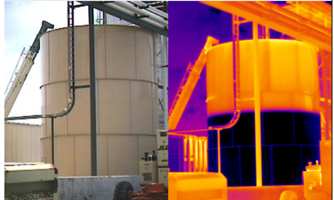
Oil and gas companies need to be able to clearly identify various levels within a tank; traditional methods are unreliable and can be dangerous, including strapping or dip-sticking.
