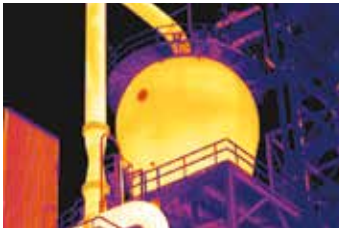
Refractory insulation inspection on a petrochemical reactor
