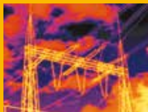
Inspection of high voltage power lines
