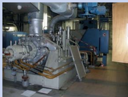
Fig. 7: Measuring device for shaft vibrations; special water pump and mounted balancing weights
