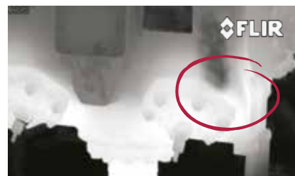
Captured gas leak.
